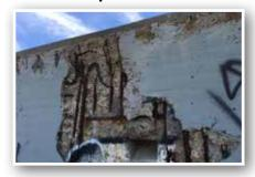
Unsound concrete removed and corrosion inhibitor applied to exposed rebar.
