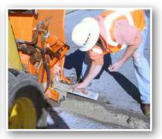
$\textit{Mixing/laying equipment can be used to lay Elephant Armor}^{\text{TM}}.$
