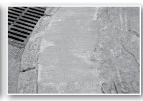
Surface was primed and Elephant Armor™ was rolled on for a permanent repair without deconstruction.
