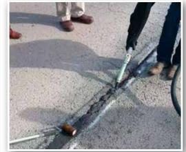
Elephant Armor™ being line-pumped into roadway micro-trench for fiber optic cable installation, using a volumetric mixer.
