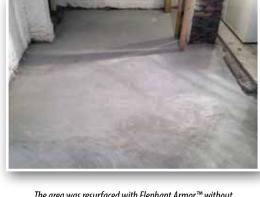
The area was resurfaced with Elephant Armor™ without deconstructing the failed surface.
