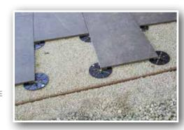
Base cross section detail using Aristokrat® Series Carrara Marble over BlackJack® BJ-4mm Pedestals
