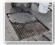
The aggregate base must be compacted and a fixed bidirectional geogrid properly installed.
