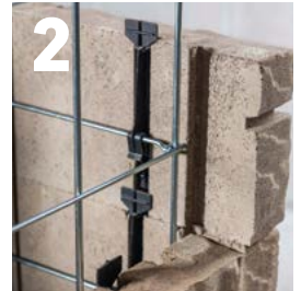
2 Use connector to attach Tandem Veneers to grid
