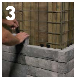
3 Attach Tandem Veneer with Connector
