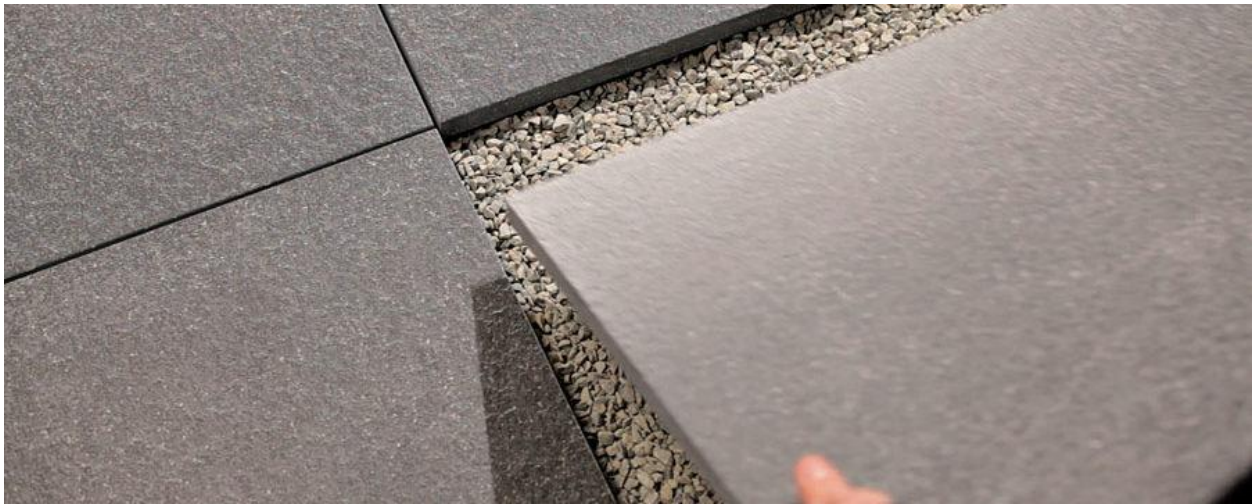
Pavers installed on screed stone
